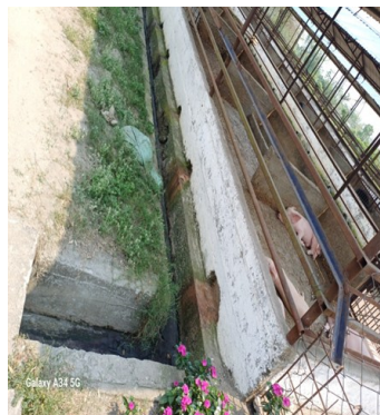
Fig. 6: Lateral view of pigsty construction
